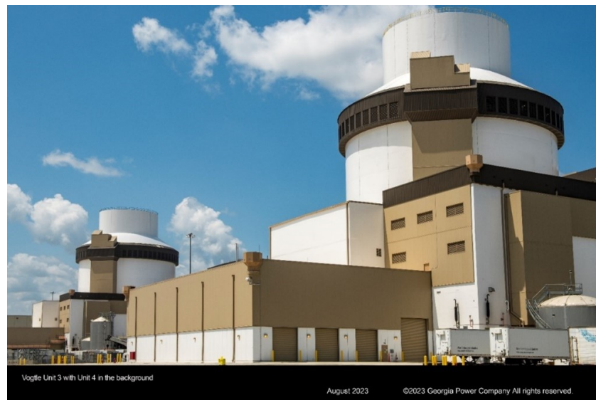
Figure 3.6 The two AP1000 units of the Vogtle Nuclear Power Plant (Image from Georgia Power Company)
